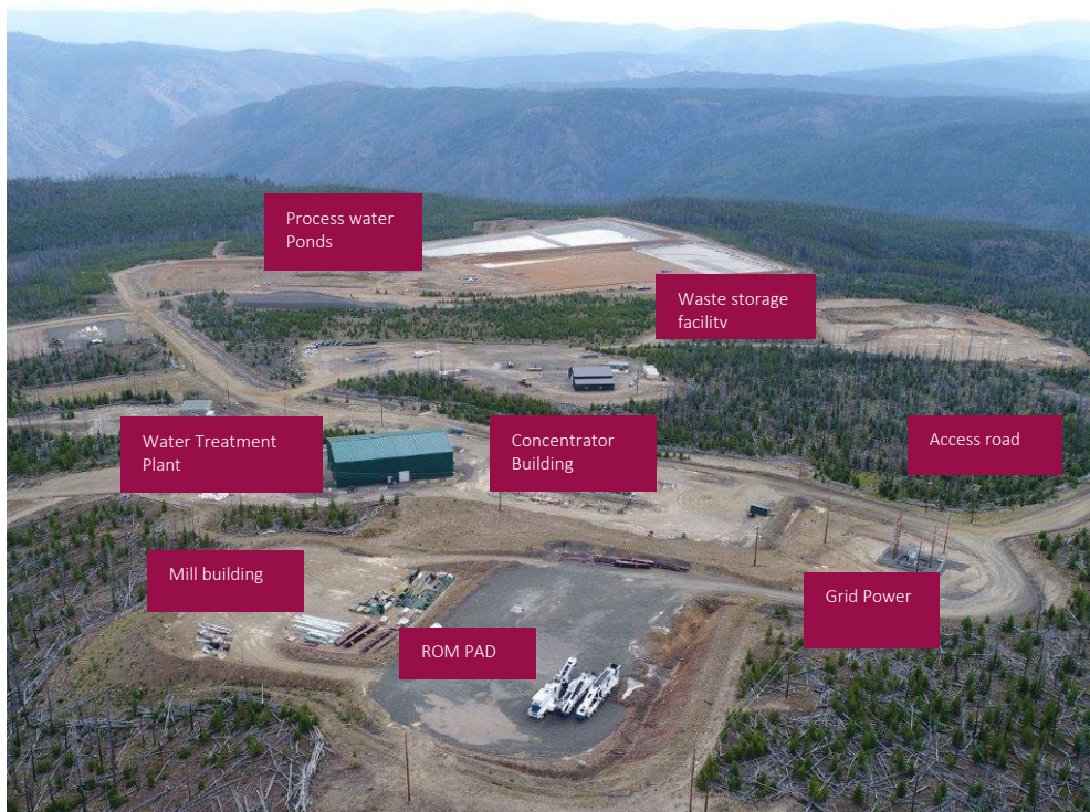
Figure 1: Current ICO Construction Site Overview
