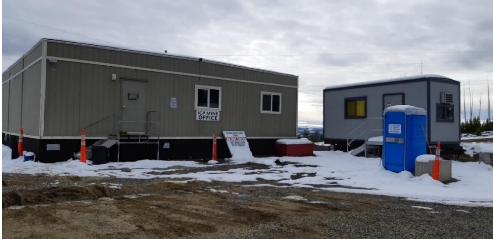
Figure 7-27: ICO Mine office
