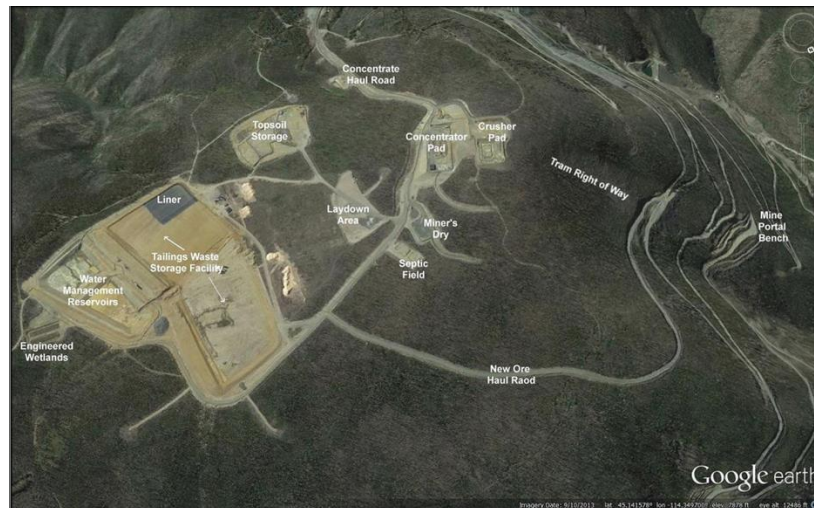
Figure 6-1: Image of ICO Showing Mill Site and Completed Earthworks after Completion of Stages I & II Construction
