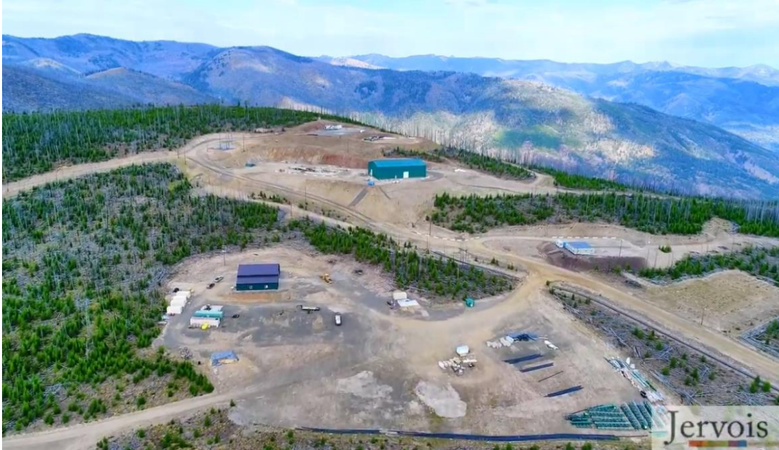
Figure 18-2: ICO Plant Infrastructure – Admin and Maintenance Buildings, Water Treatment Plant
