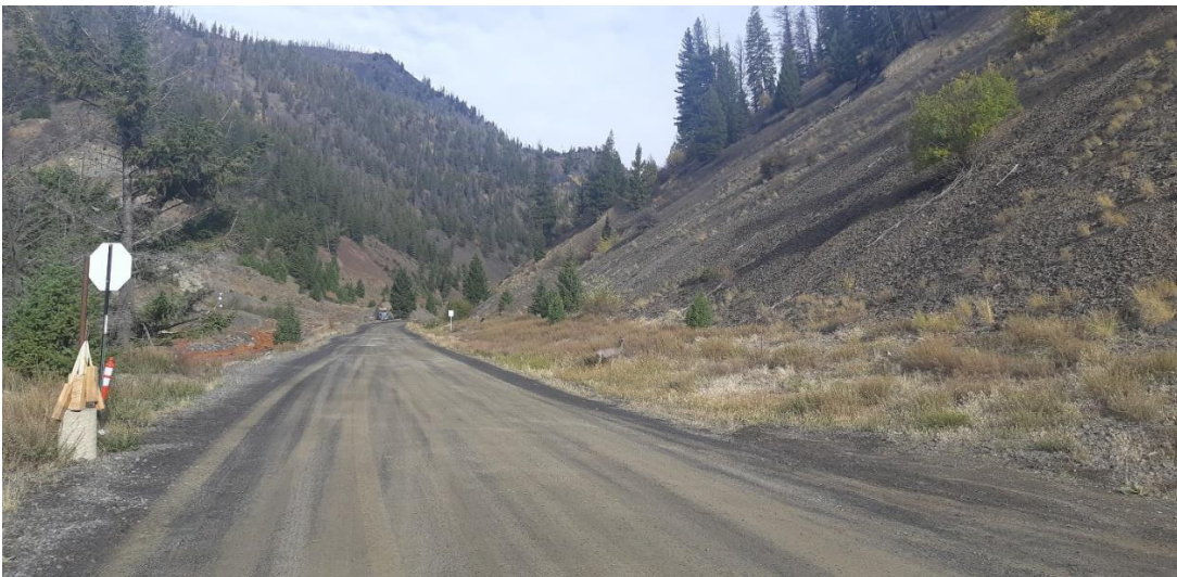
Figure 7-26: Gravel Access Road to Site
