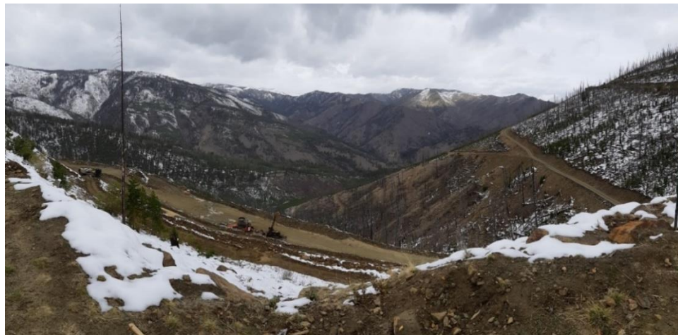
Figure 7-31: Active Drilling and Access Roads
